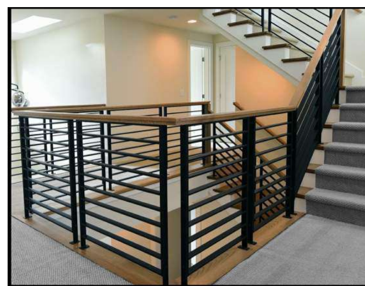
1 METAL PIPED GUARDRAIL
